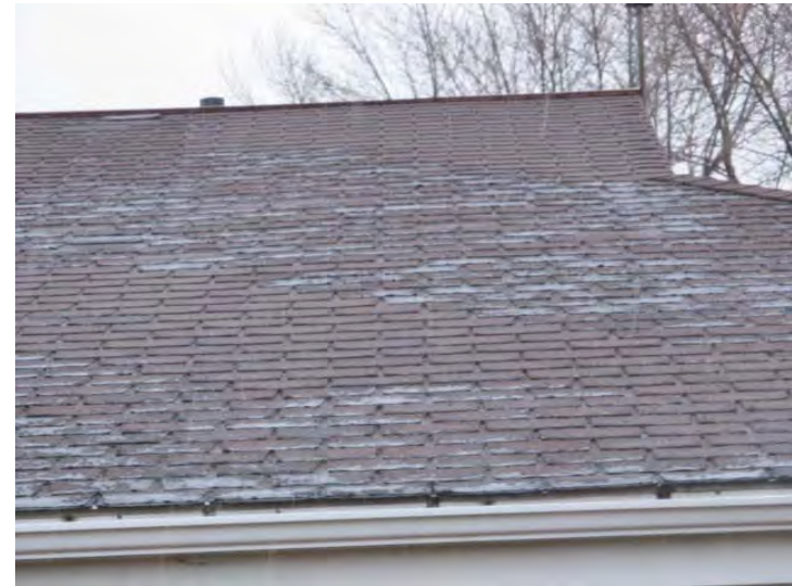
Asphalt shingles on roof surfaces have exceeded their service lives and are in poor condition throughout the development
