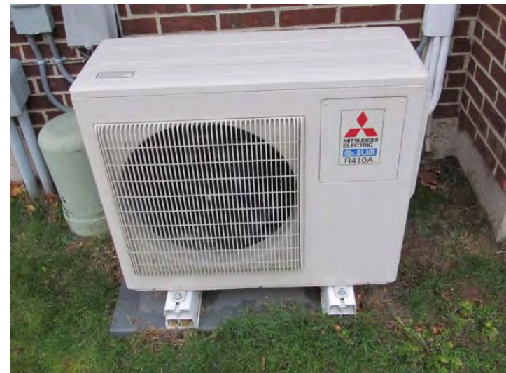
Typical exterior-mounted condenser found at each unit for recently installed heat pumps
