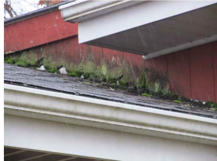
Wood siding exhibits deterioration – This view in area between roof levels of building set into slope
