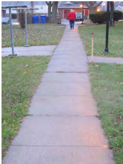
Typical concrete walkway – Isolated cracks, minor displacement and potential trip hazards noted
