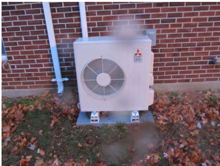
Recently installed condenser unit for heat pump serving interior spaces at Community Building
