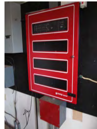
Original zone-type fire alarm control panel located at Community Building
