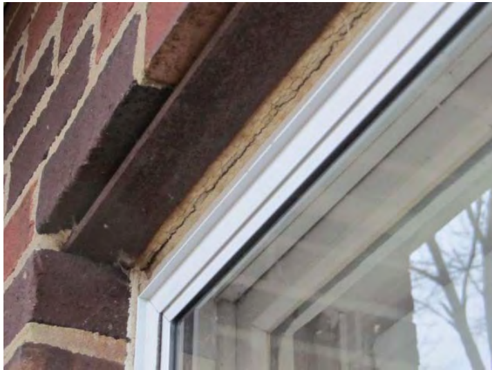
Steel lintels in need of surface preparation and painting and perimeter caulking in need of replacement
